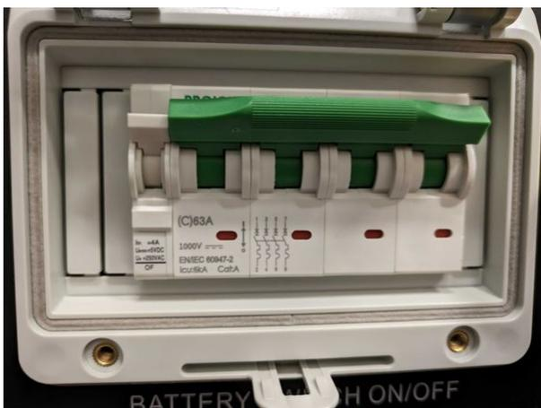
Batterieschalter (Battery Switch On/Off)
